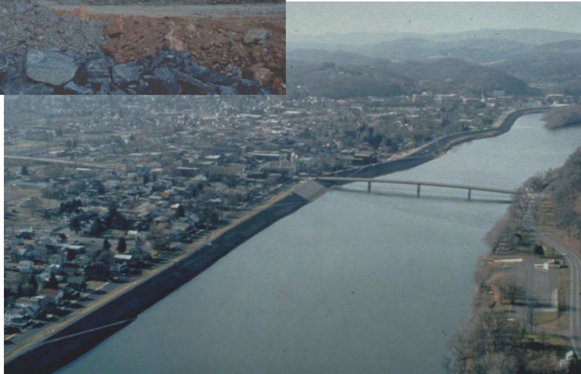
Flood Protection Levee Lock Haven, PA
